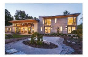
says. The pavilion roofs appear to be flat, but the center actually slopes in (the inverse of a typical New England roof, where the center is the highest point) to channel rainwater toward a cistern filled with river rocks below. During storms, it creates a picturesque waterfall outside the hallway windows.
